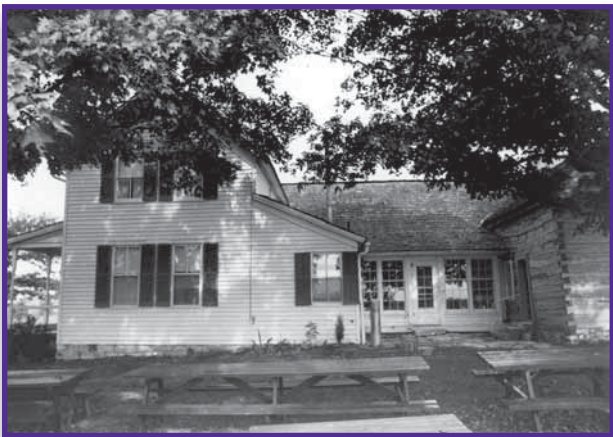
Bergt Farm Complex Missouri State Archives, Dept. of Natural Resources, National Register of Historic Places Nomination Files
