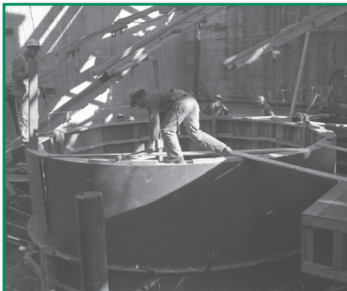
Unit 7 Pit Liner Form, 1952 [from later additions to Bagnell Dam] Bagnell Dam Construction Photographs, Missouri State Archives
